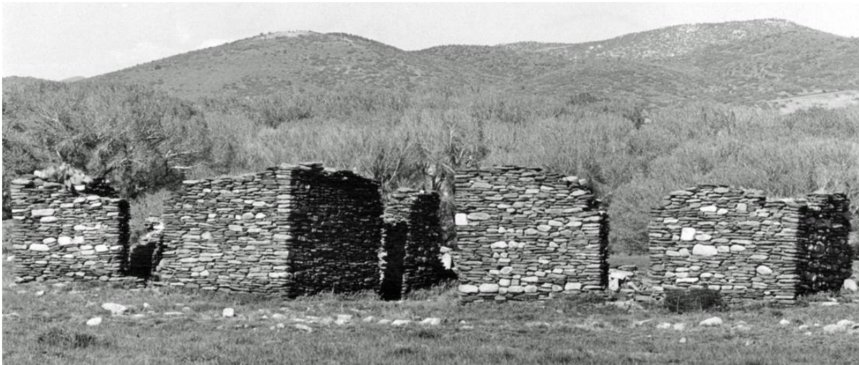
Agua Caliente Ranch as it appears today Photo courtesy of Marshall Trimble
